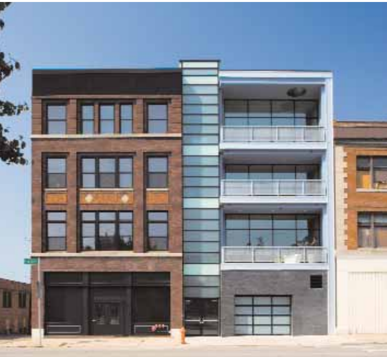
Parabuildings can double the size of the original building and provide equal yet contrasting structures. The four-story, modern glass and steel addition to a four-story, historic brick building, formerly home to a printing company at the turn of the last century, now houses 225 N. Fourth Lofts, a residential loft project with full-width terraces providing views of downtown Columbus, Ohio.
